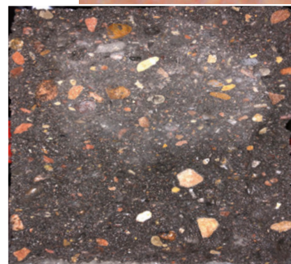
Without waterproofing admixture
